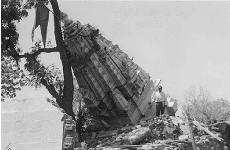
Figure 10 Overturned object at Adhoi (23.4°N, 70.5°E). (b/h) = 0.61 .
