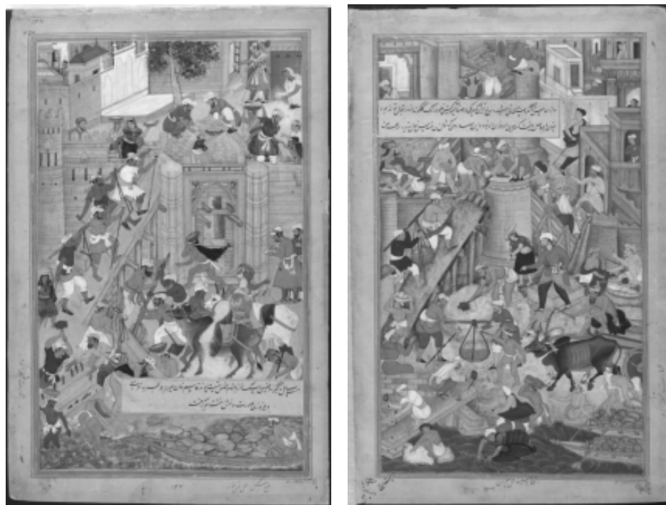
Fig. 1. (a) and (b) Miniature paintings from Ākbarnāmā showing the construction of Agra fort 18,19 .
