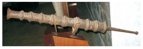
Fig. 11. Forge welded cannon at Tripura State Museum
