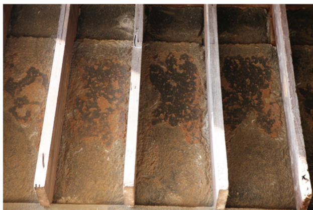
Fig. 3. Photograph showing two layers of mud plaster at Bhaja
