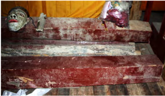
Figure 12 Beam of assembly hall.
