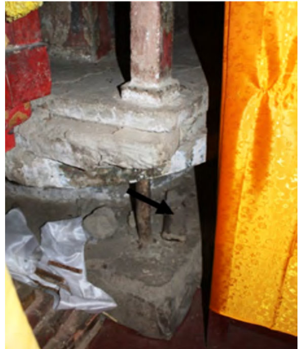
Figure 18 Wood sample from the base of wooden framework of main deity (arrow).
