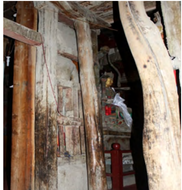
Figure 17 New pillar of Assembly hall.
