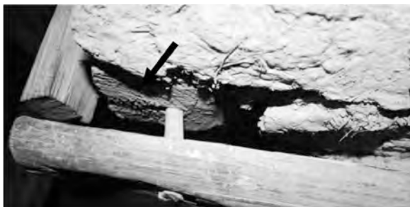
Figure 5 Wooden nail used in the wooden framework of main deity (arrow).
